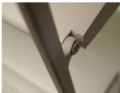
Clearview Tilt Rod screw & louvre notch
